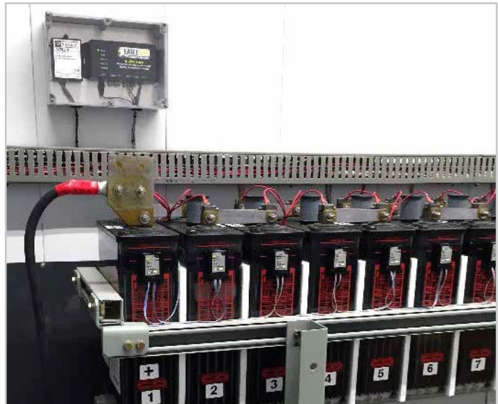
Installation to Battery Cells
