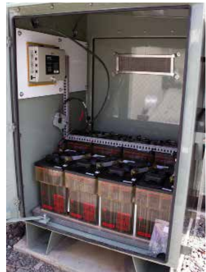
Installation to 48V Switchyard Battery
